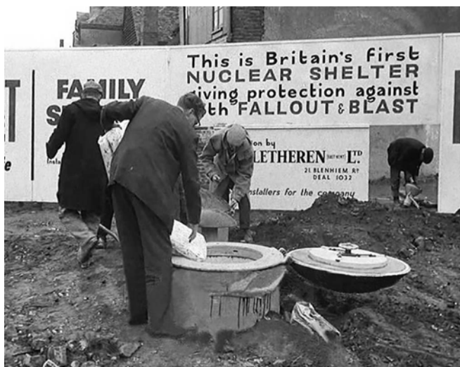
Lowering the bedding into the shelter
